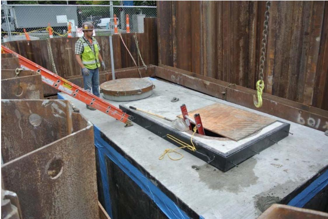
*Installation of a vault that houses electrical and fiber-optic wiring between Seneca and Spring streets.*
