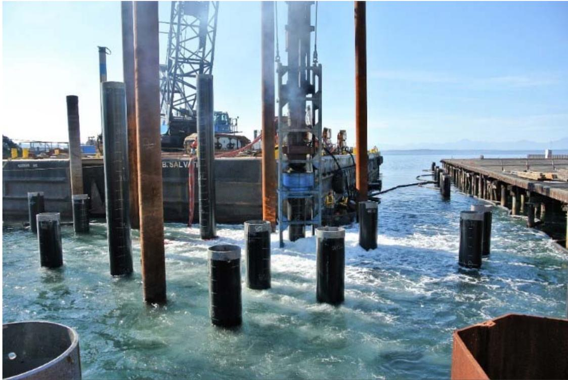
*The bubble curtain around new steel piles helps protect aquatic life during construction.*
