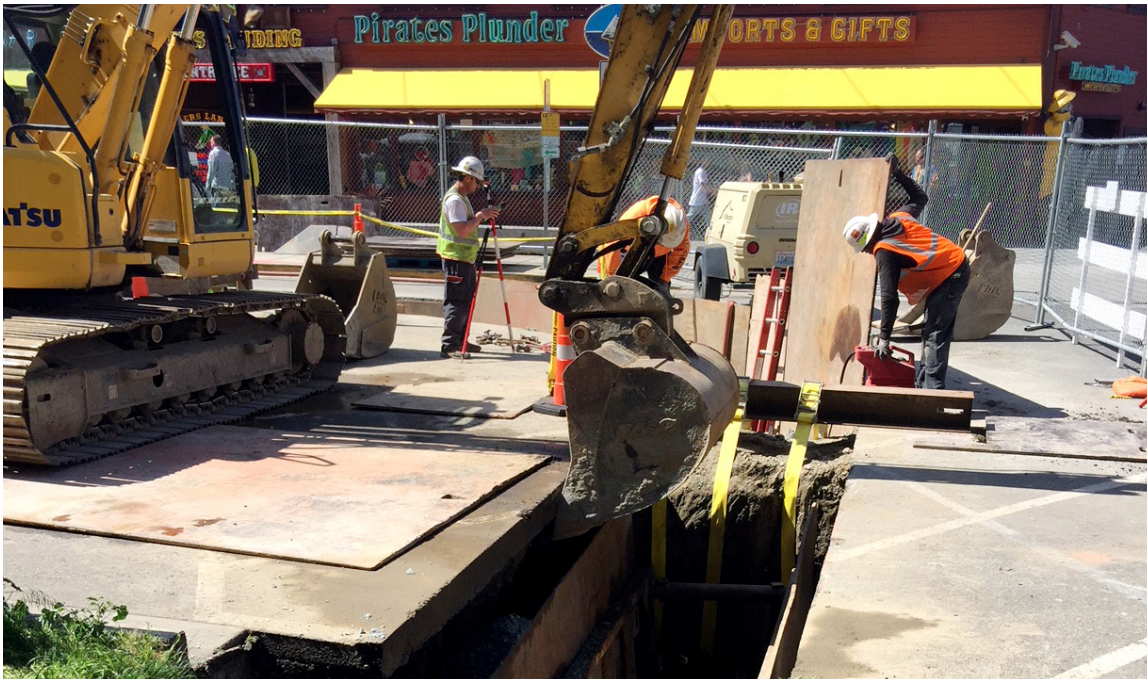
Digging trench for duct bank installment
