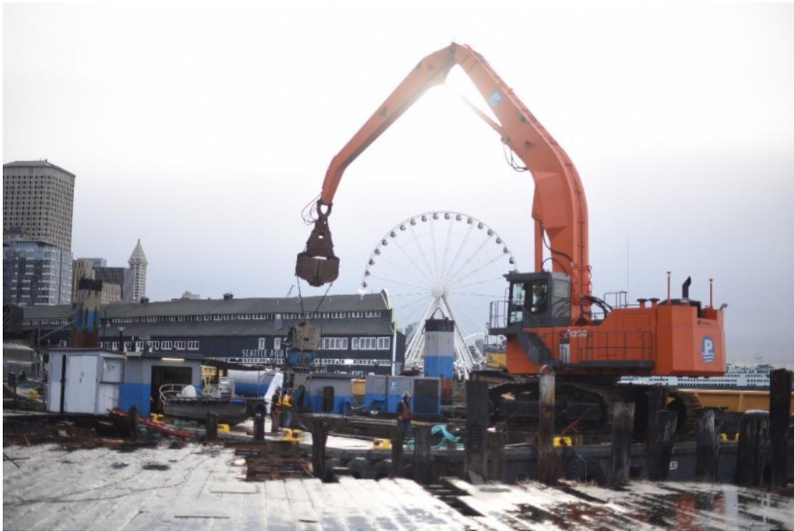
*Crews remove the aging deck and pilings from Pier 62.*
