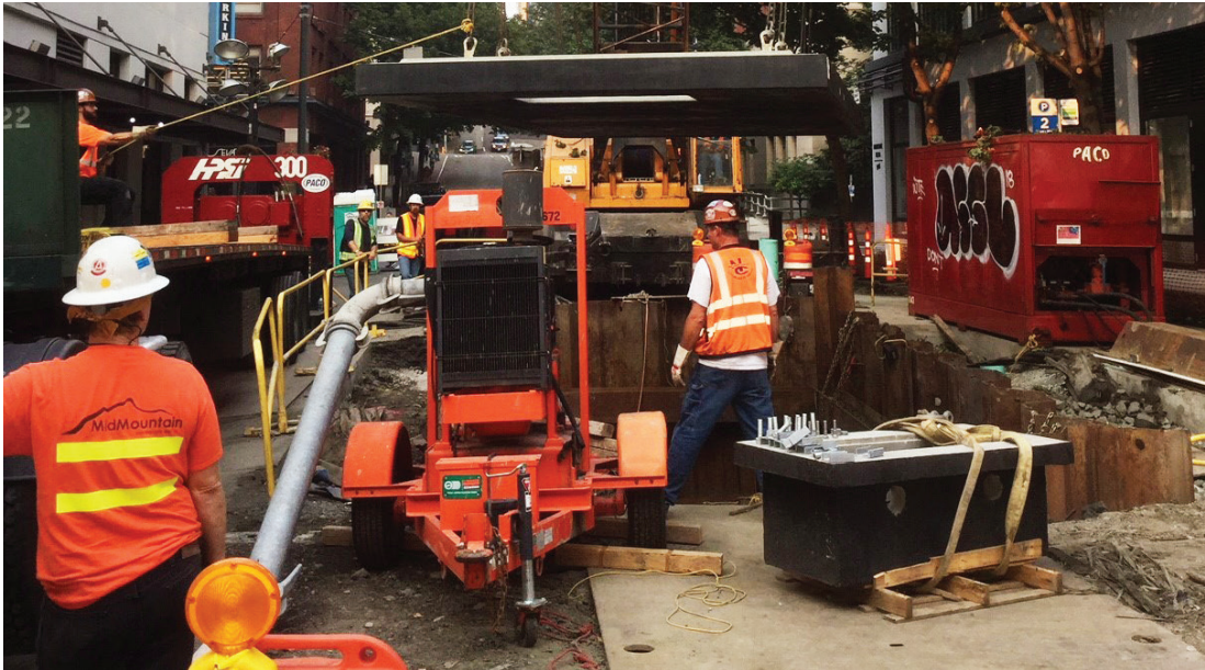
Example of vault installation work
